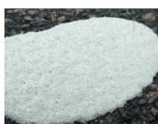
7) Inspect bonding with chisel and hammer. If correctly applied parts of the asphalt surface layer will break off together with the MeltMark®. If not proper bonding repeat heating process or consider if surface preparation has to be improved.
